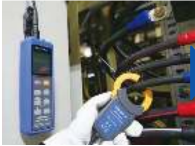
Connect the sensor to the Display Unit CM7291 and clamp in around the cable to be measured.
