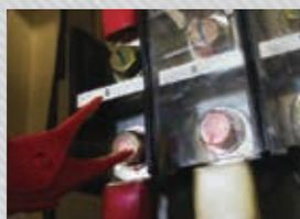
The CM3286 can safely measure service wires with a wire-to-ground voltage of up to 600 V as well as wires found in distribution panels. The clamp meters also feature a safe design that can withstand a transient overvoltage of 8 kV in case of a lightning strike.
