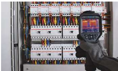
Electric Panel Inspection
