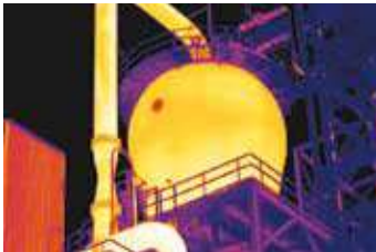
Refractory insulation inspection on a petrochemical reactor
