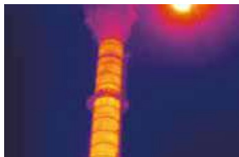
Refractory material inspection on a furnace chimney.
