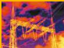
Inspection of high voltage power lines
