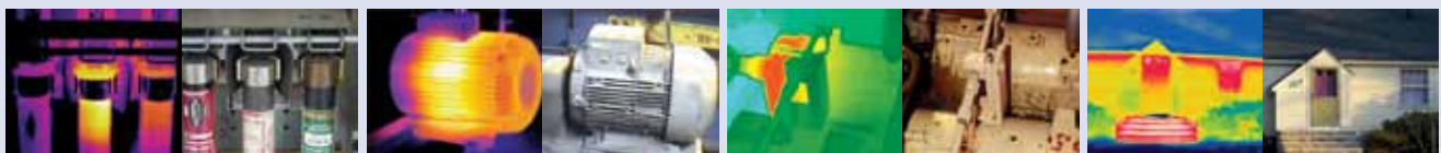
Electrical: Hot Fuses
